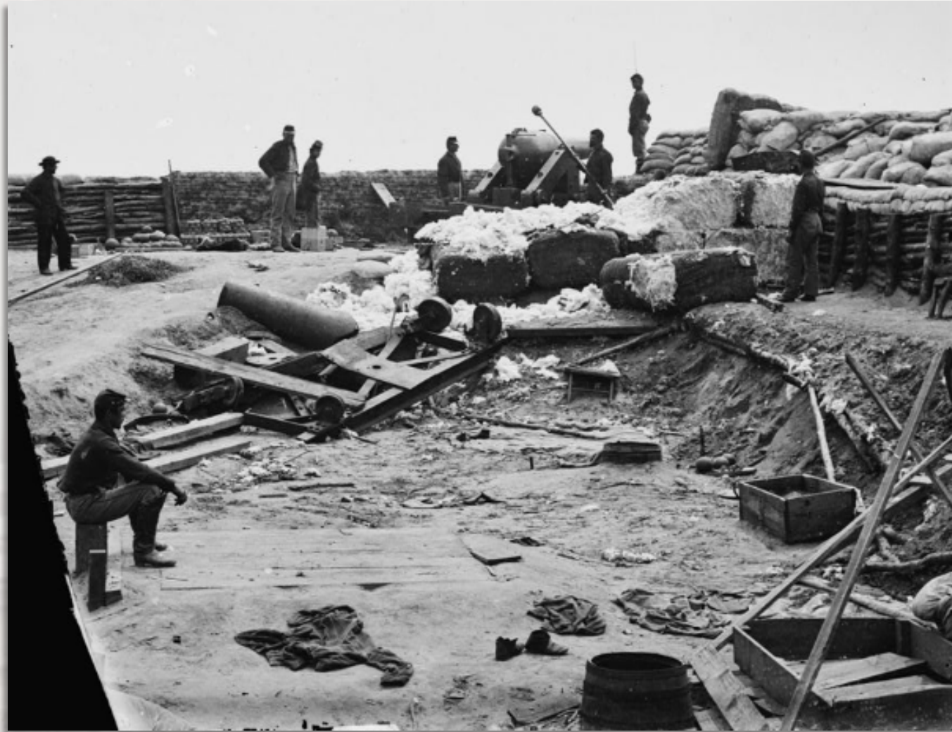
Confederate fortifications reinforced with bales of cotton The Library of Congress
