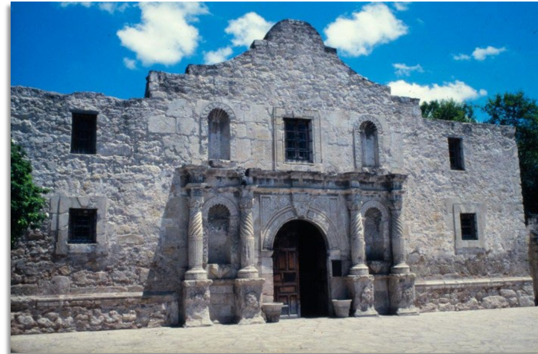
Mission San Antonio de Valero Founded in 1718 in San Antonio The Portal to Texas History The University of North Texas
